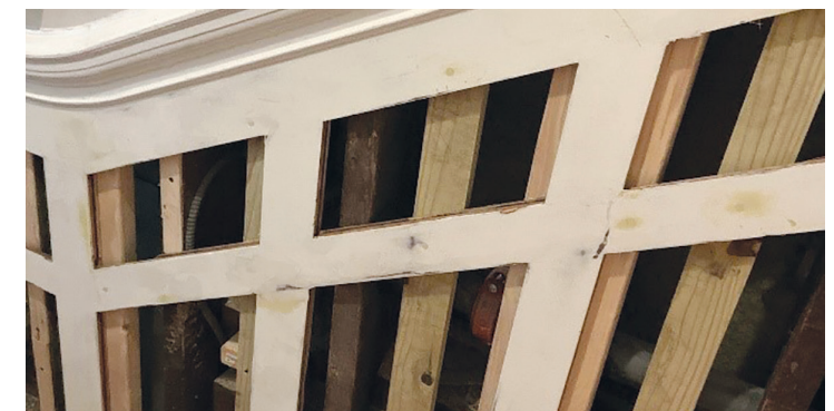
Panels removed with backing installed.
